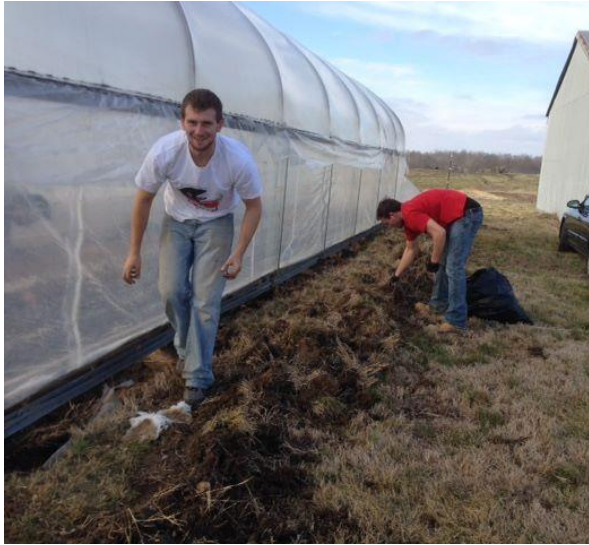
Digging out for the bamboo barrier
