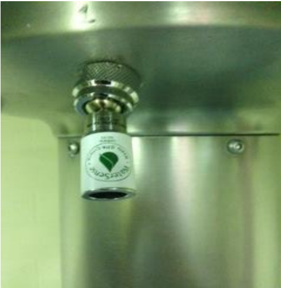
Actual shower head photo from Recreation Center Men's Locker room shower.
