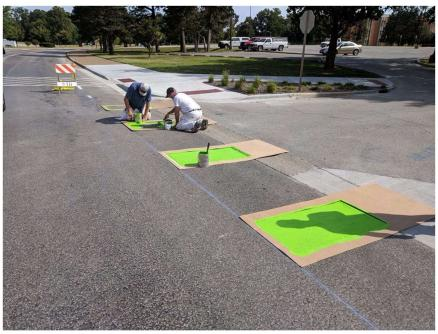
• Image 1: This image portrays work being done to complete the "green junctions" (perpendicular vehicle crossing) on the bike lanes.
