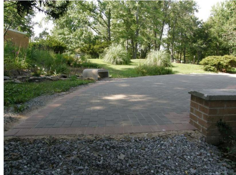
Figure 2. Patio on east side of the Agriculture building constructed of recycled fly ash bricks.
